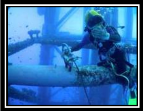
Diver carrying out MPI Inspection
